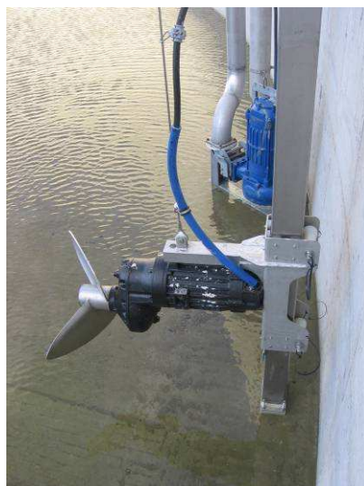
Figure 7.22 Submersible motor propeller stirrer (AGRINZ 2006)
