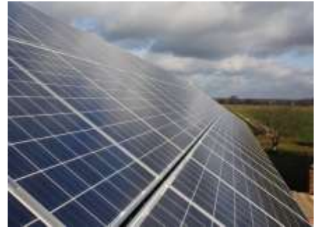
Figure 6: Crystalline Silicon PV array
