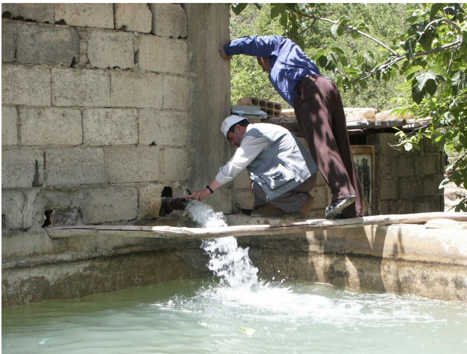
Groundwater pumping and short-term storage
