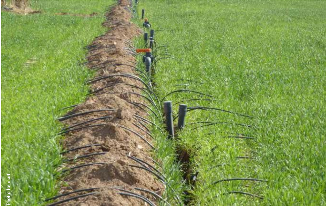
Installation of a drip irrigation system (Source: Lennart Woltering)
