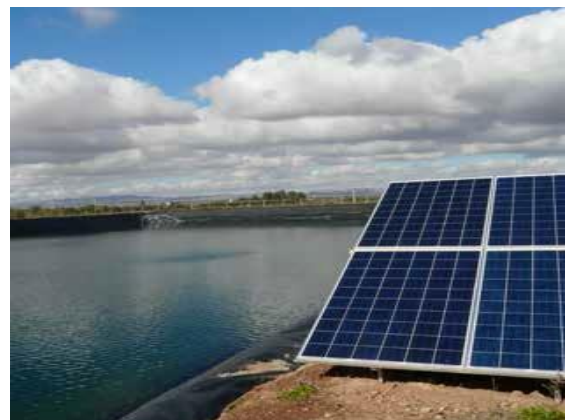
Open plastic foil-lined reservoir
