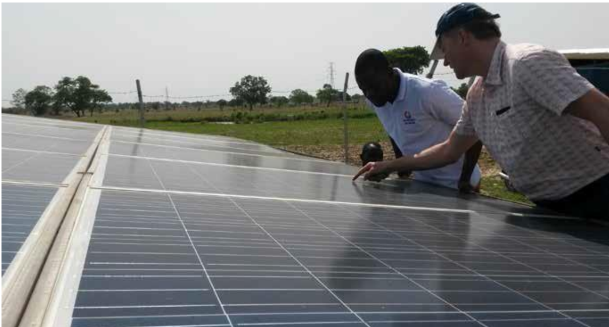
Visual check of the solar panels
