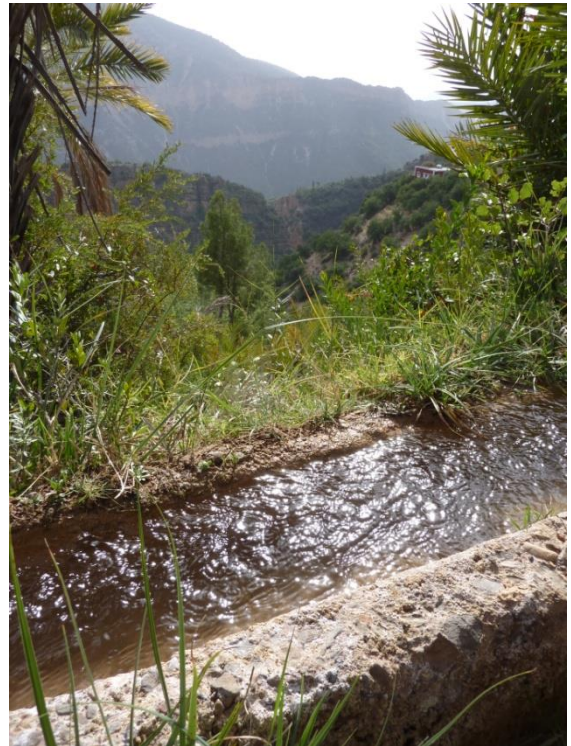
Concrete irrigation canal
