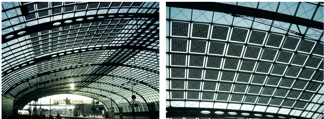
Figure 3: Semi transparent solar PV roof at the main station of Berlin/Germany
